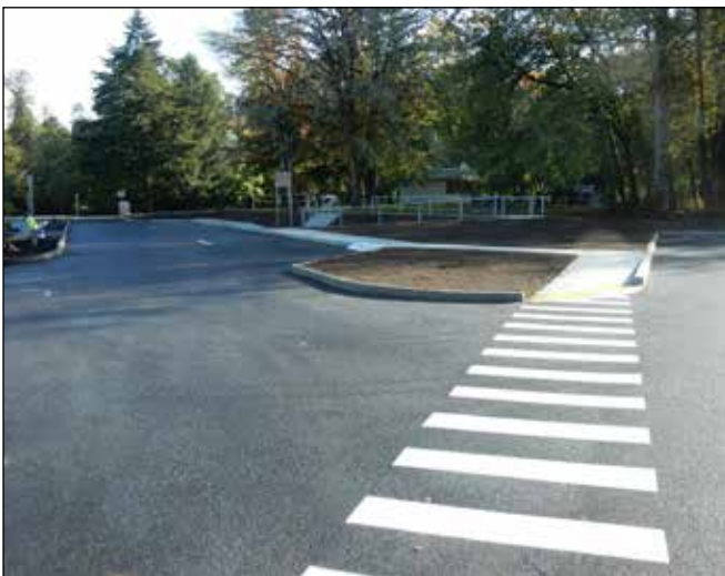
Newly Constructed Walkway to Hendricks Bridge Boat Ramp (East Viewpoint)
