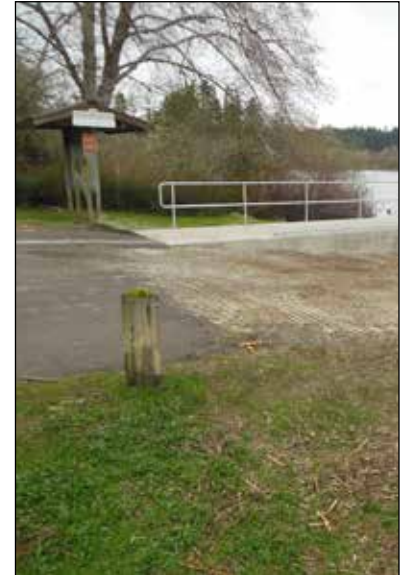
Boat Ramp & Fishing Pier, Westlake County Park
