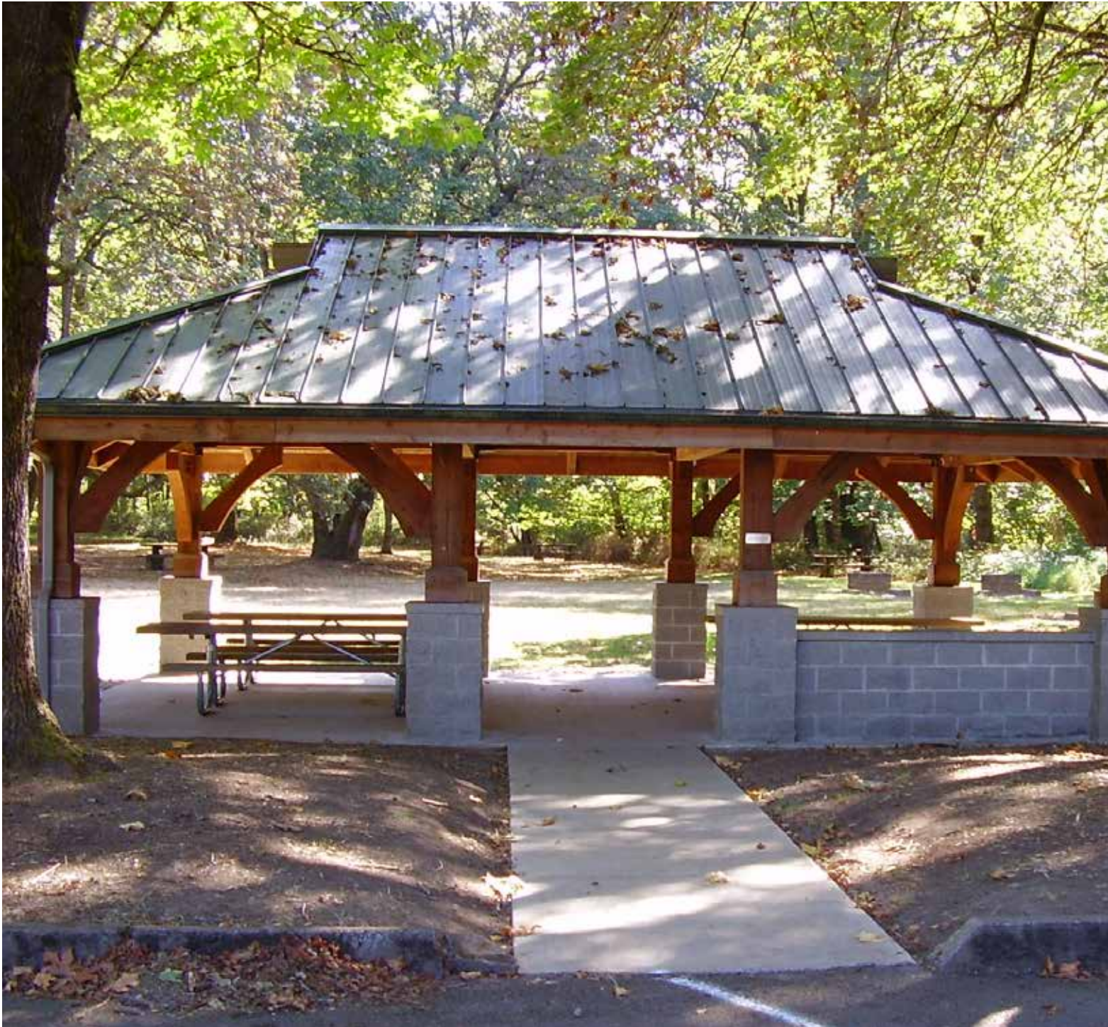
Picnic Shelter at Hendricks Bridge County Park
